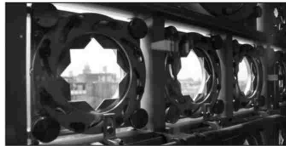
Figure 35: Mechanical system for dynamic screen
