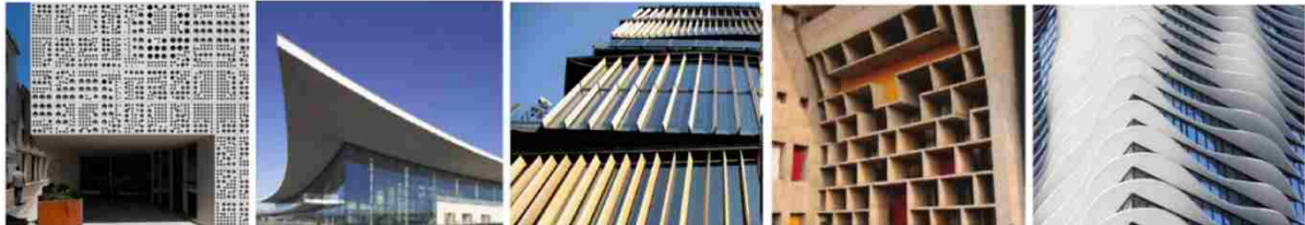
Figure 11: From left to right: Overhang-Gibraltar Airport by Blur Architecture and 3DReid, Louvers- Aqua was designed by Jeanne Gang, Fins-Asakusa Culture Tourist Information Center, Eggcrate-The Chandigarh High Court, Perforated Screen- Social Facilities in Roses by Exe architectura.
